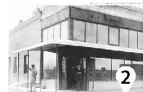
Willard Bank Building
